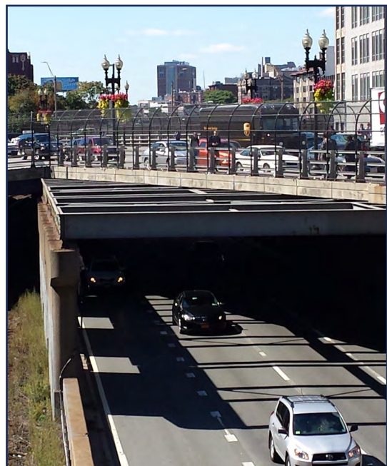
Figure 27: An example of a partially constructed decking over a highway in Boston's Back Bay. Photo Credit: John Gravelin.
