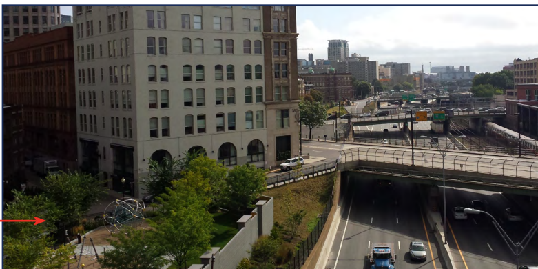
Figure 25: Trees, wall barriers and other vegetation may reduce exposure from this playground directly next to this highway - a particularly vulnerable place for children. Photo Credit: John Gravelin.
