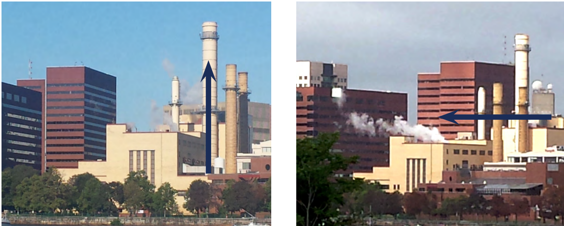
Figure 9: These images illustrate the effect of wind speed on pollution mixing. Left: Low wind speed results in little mixing near the stack. Right: High wind speed causes greater mixing near the stack. Photo Credits: John Gravelin.
